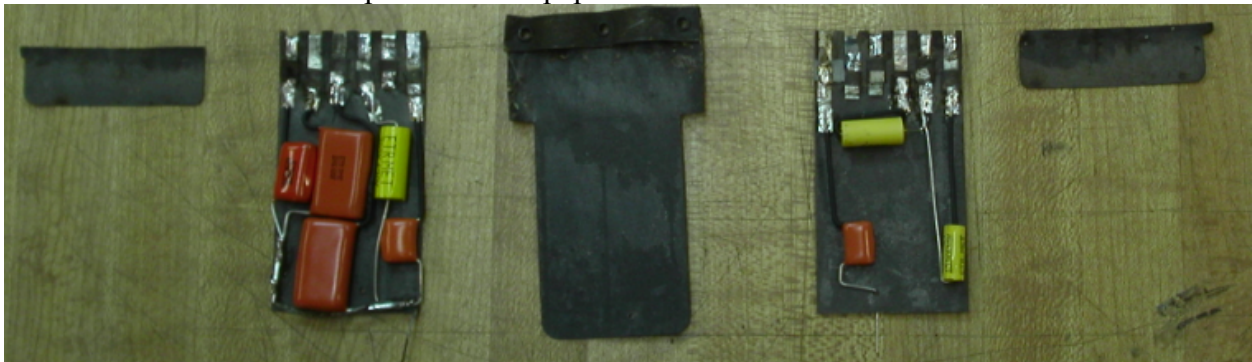
New Bypass Capacitors Installed
