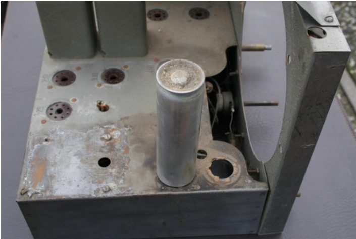
Missing PWR Transformer
