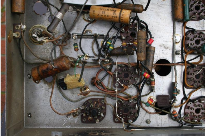
Cut Wires Under Chassis
