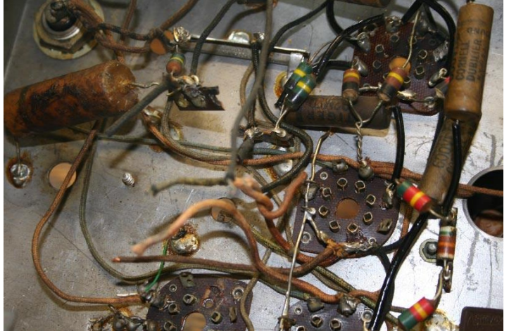
Cut Wires Under Chassis
