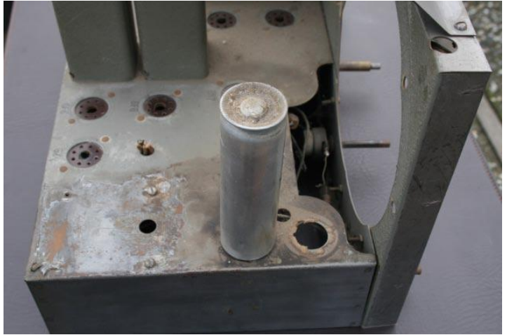
No PWR Transformer - Missing Cap
