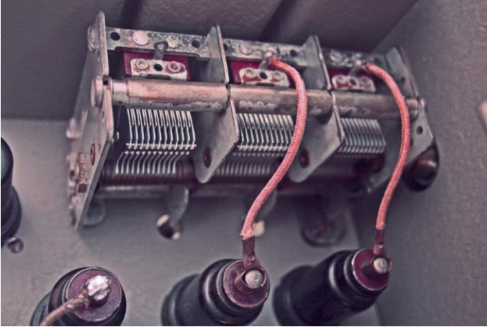
Cleaned Capacitor Installed
