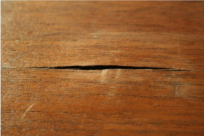
Cabinet Top Veneer Damage
